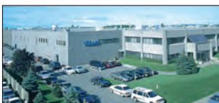
Montreal, Canada Velan Inc., Plant 2 and 7
