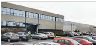
Montreal, Canada Velan Inc., Plant 1 and 5
